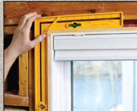
Accurately install windows and doors
