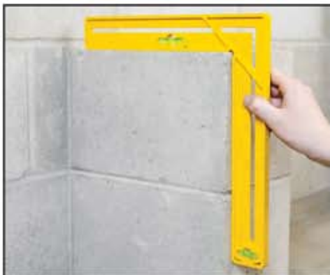
Precisely lay masonry for foundations
