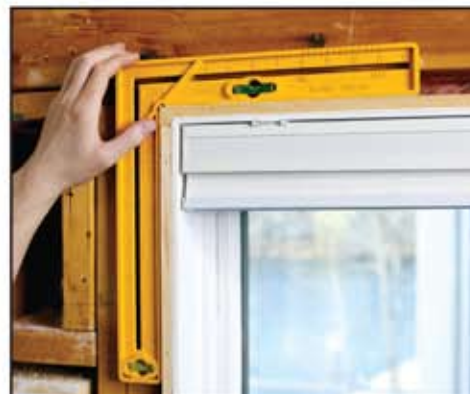
Accurately install windows and doors
